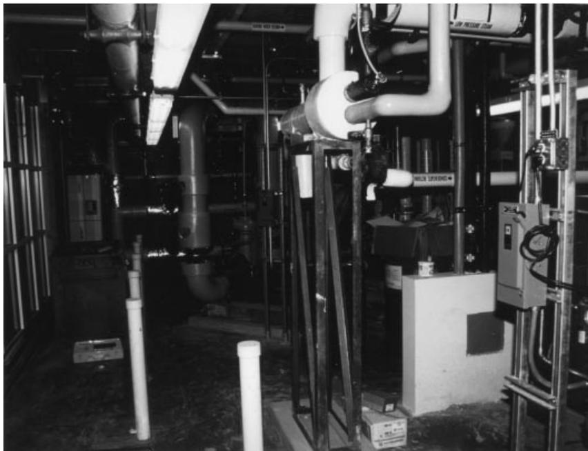
Fig. 6. Exposed features of the building demonstrate how buildings function. In this case, the mechanical room is exposed, with color-coded piping.
