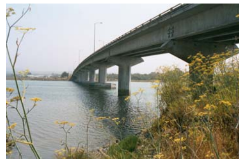
Figure 6. Humboldt Bay Bridge (G. Deierlein photo).
